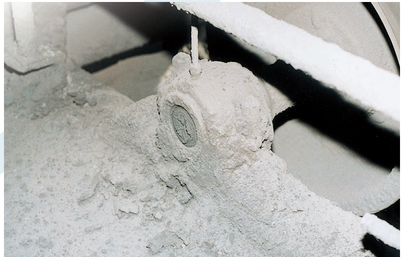
Plummer block usage condition
